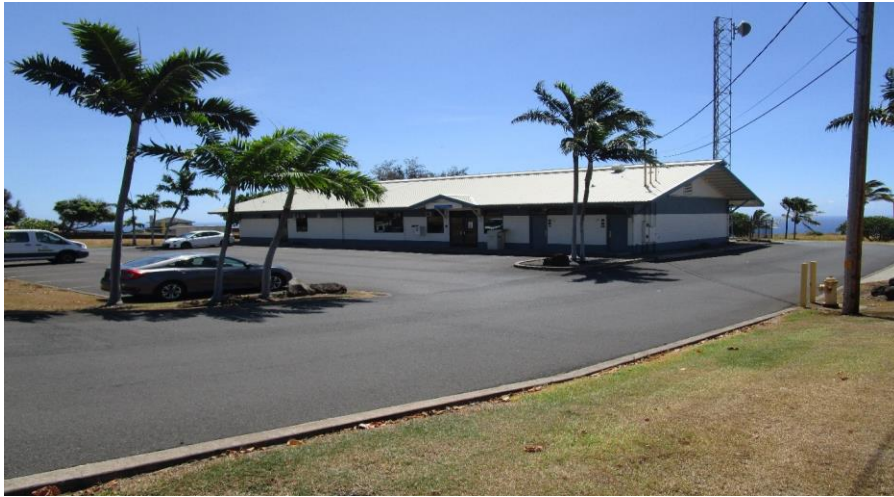
KA' Ū POLICE STATION
