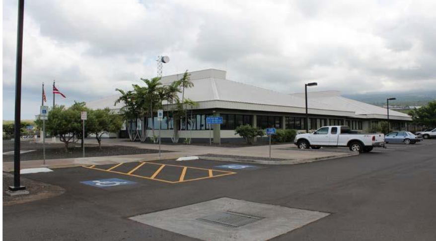
KEALAKEHE POLICE STATION 74-611 Hale Maka'i Place, Kailua-Kona, Hawaii
