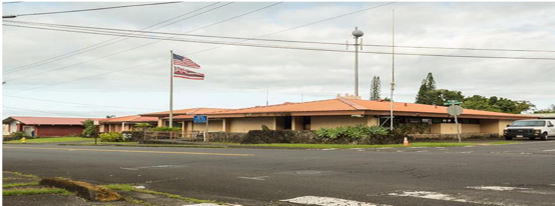
Photo of the Kea'au Substation
