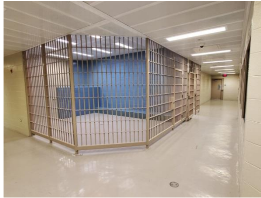
Photo above depicts the large holding cells in the East Hawaii Detention Facility
