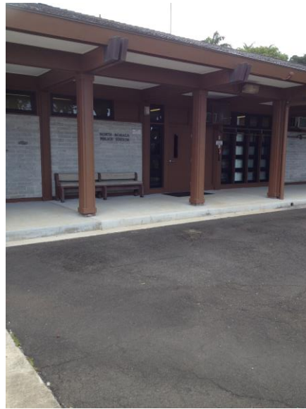
North Kohala Police Station
