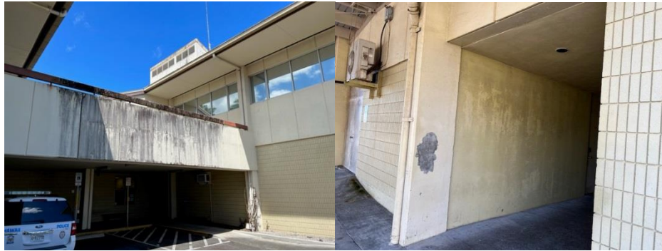
Exterior views of the South Hilo Police Station
